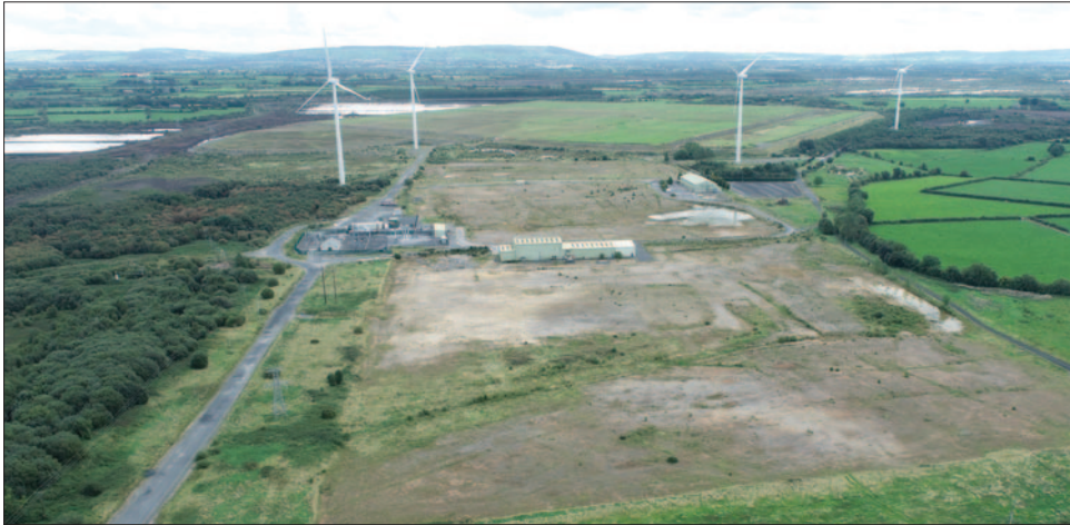
Lisheen Mines Redevelopment, Courtesy Tipperary County Council
